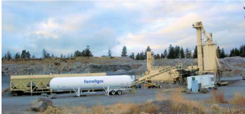
Figure 8: Propane Trailer in front of a portable asphalt plant
