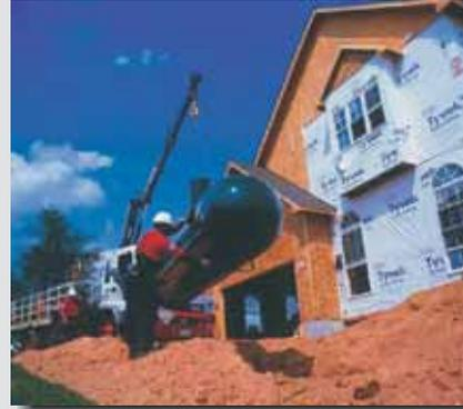
Failure to provide proper [tank] protection can cause hidden corrosion and potential leaks as well as weakening of the tank wall over a period of time.
