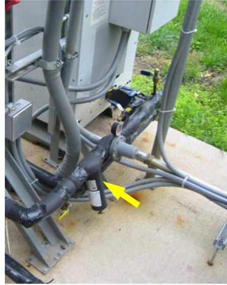
Figure 10. MT coalescing filter
