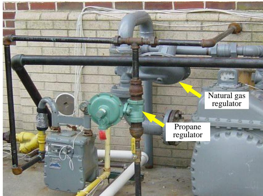
Figure 11. Natural gas regulator and propane regulator
