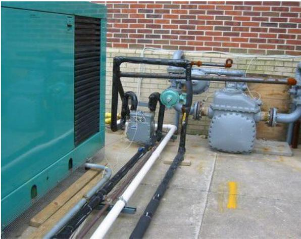
Figure 5. Heat trace and insulation applied on propane pipes
