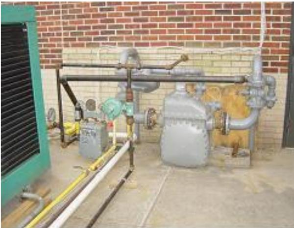
Figure 6. Piping, gas meter and emergency generator (left front green one)
