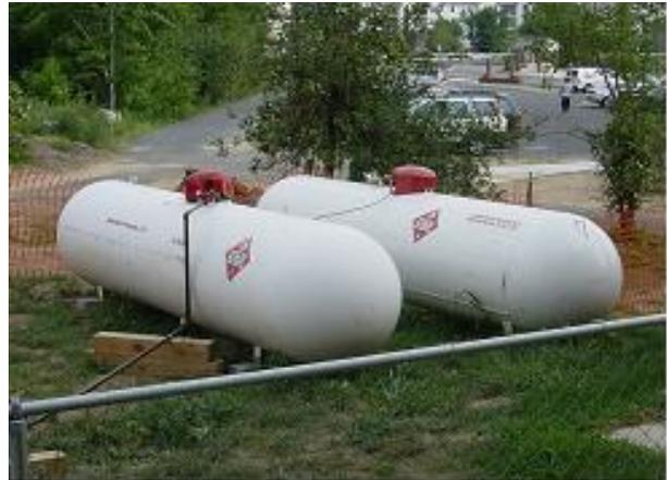
Figure 4. Two 1000-gallon propane tanks
