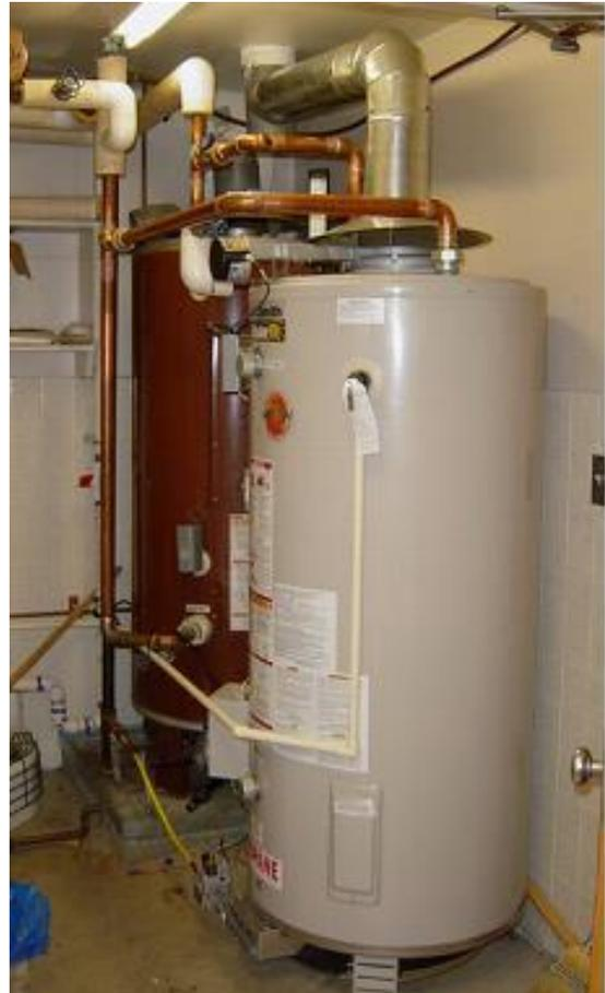
Figure 7. New domestic hot water heater tank burning on propane
